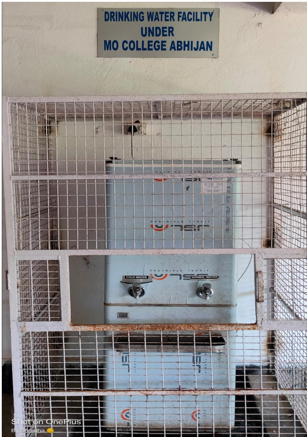
Drinking water facility
