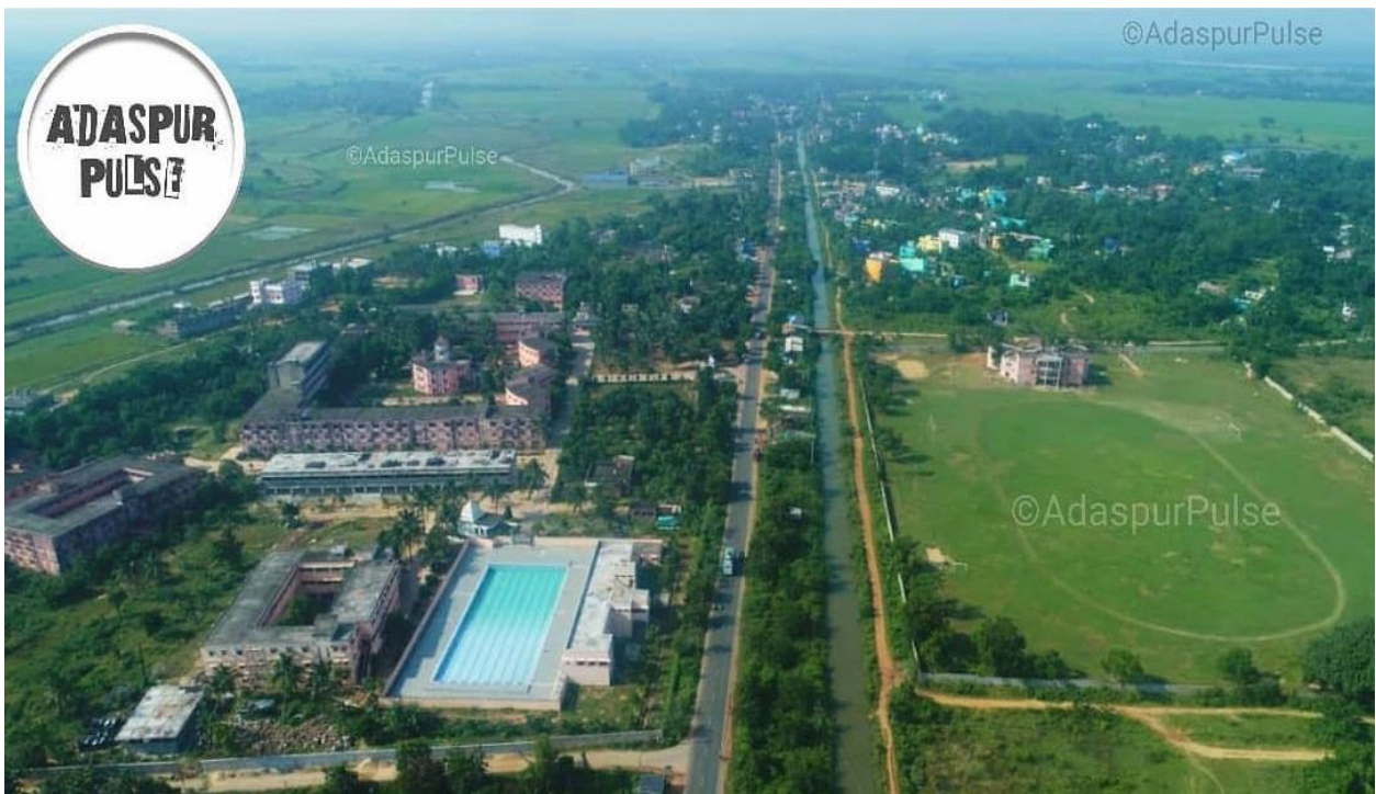
Aerial View of the College
