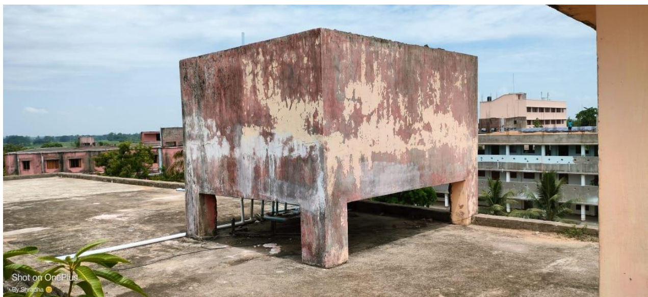
RCC Tank in Science block
