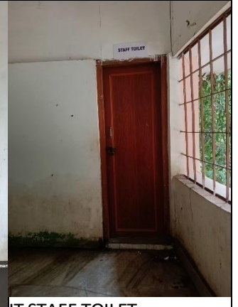
IT STAFF TOILET
